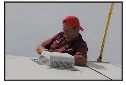
Here is Shannon cutting the membrane and placing one of the roof vents in place. They then added a layer of membrane around the edges and those were also heat welded to seal them.
