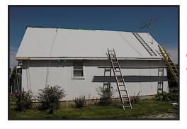
Not sure if you can see it, but just to the left of the rope hanging down (above the butterfly bushes) there is glue that needs cleaning off before the rails are applied. I only point this out because this is common and they have a solvent to remove it.
