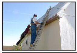
There was minor damage along the soffit (that is the wood perpendicular to the wall under each overhang) each place they used the angle iron to 'pop out' the old fascia. But it was easily caulked during the painting prep.
