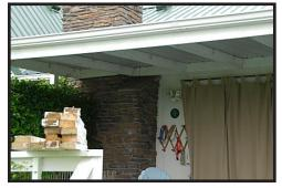
During the first rain delay, the crew started the process of 'beefing up' the roof of the back porch. We discovered that the beams were about 3 feet apart and that is not adequate for the crew to be walking on top of (for one thing).
