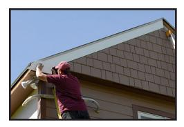
This gable is on the north side and it gets beaten on by wind and rain in the winter. The cementatious fiber siding and AZEK boards will make a tremendous difference!
