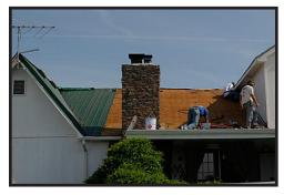
Finally, they get to start on the back. But this area is very important to get right because of the chimney and the flashing that needs to keep the water away from it.
