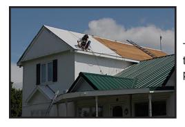
This day turned out to be windy, which slowed progress tremendously, so they welded each section as they went to avoid potential wind problems.
