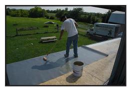
Now, this is the usual application for a single-ply membrane: on a no/low-slope roof. So this section went very quickly.
