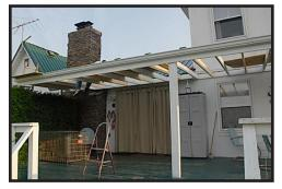
The back porch had to be reinforced (as mentioned previously) before they could work on the the back side of the house. So you can see the new beams here.
