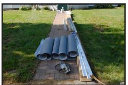
The membrane comes in rolls that are cut to size on the ground and then carried to the roof as needed. (The gray you see in the picture is actually the back of the product.)
