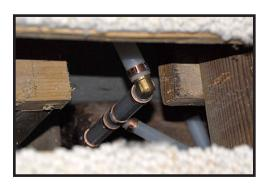
The water comes into the house in the master bedroom and there is a mock-register opening that allows access to it. The water for the master bathroom splits off before it continues into the basement. So there is now a regulator installed at this location as well as a shut off for just the master bathroom. The shut off for the rest of the house is in the basement.
