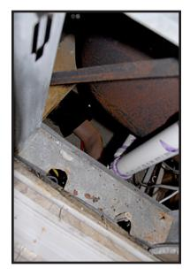
Here is proof that Cody fit in the crawlspace - that is his arm. He is running the new PEX and pulling out the old polybutylene.
