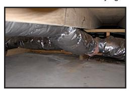
the ductwork as it came in from the basement access (about 1/2 way between the south and north walls) running from east to west and where the 1st "T" divides the run to run north (for 2 registers) and south (for 1 register). FYI, it is placed along side a framed wall in the center of the space that supports the floor joists).
