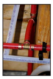
Here is a close-up of the PEX... red is for hot water, white is for cold.
