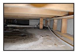
the water line where it meets the PRV (behind the vertical board, in front of the concrete hip wall).
