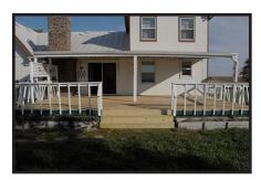
We rented a floor sander and the hubby used it to remove "cupping" on some of the boards. In case you are not familiar with that word, it describes a board that has bowed so that the edges are higher than the middle which makes it retain water longer.
