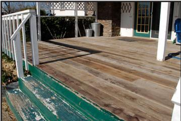
All the boards are now replaced and fastened! The hubby decided that a couple of the boards were too close together in spots (due to warping primarily) and used the circular saw to remove those bits.
